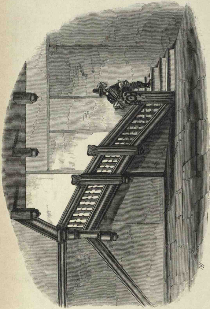
STAIRCASE, PEEL HALL, CHESHIRE.
